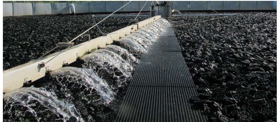
Trickling filters
